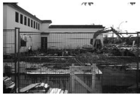
Laying the foundation.
